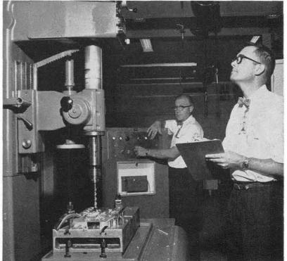
EVALUATING a numerically controlled drilling machine are E. S. Roth (foreground) and A. R. Konecny of Advanced Manufacturing Development Section 2564-1. The machine is automatically controlled by the computer-like console operated here by Konecny.
